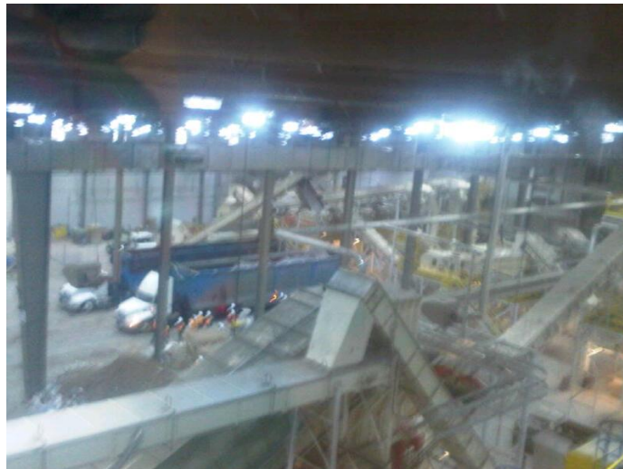
Figure 5: Materials recovery facility (MRF) at EWMC
