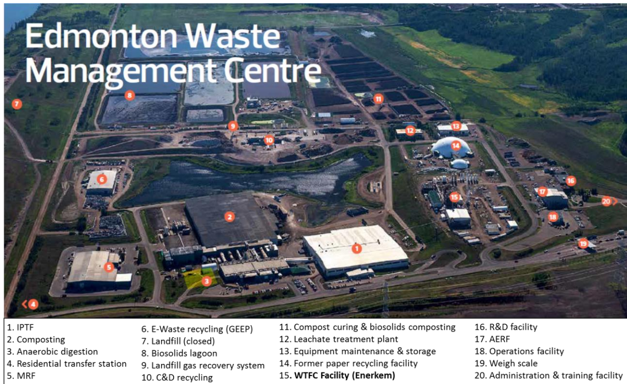
Figure 3: City of Edmonton Waste Management Centre (EWMC)
